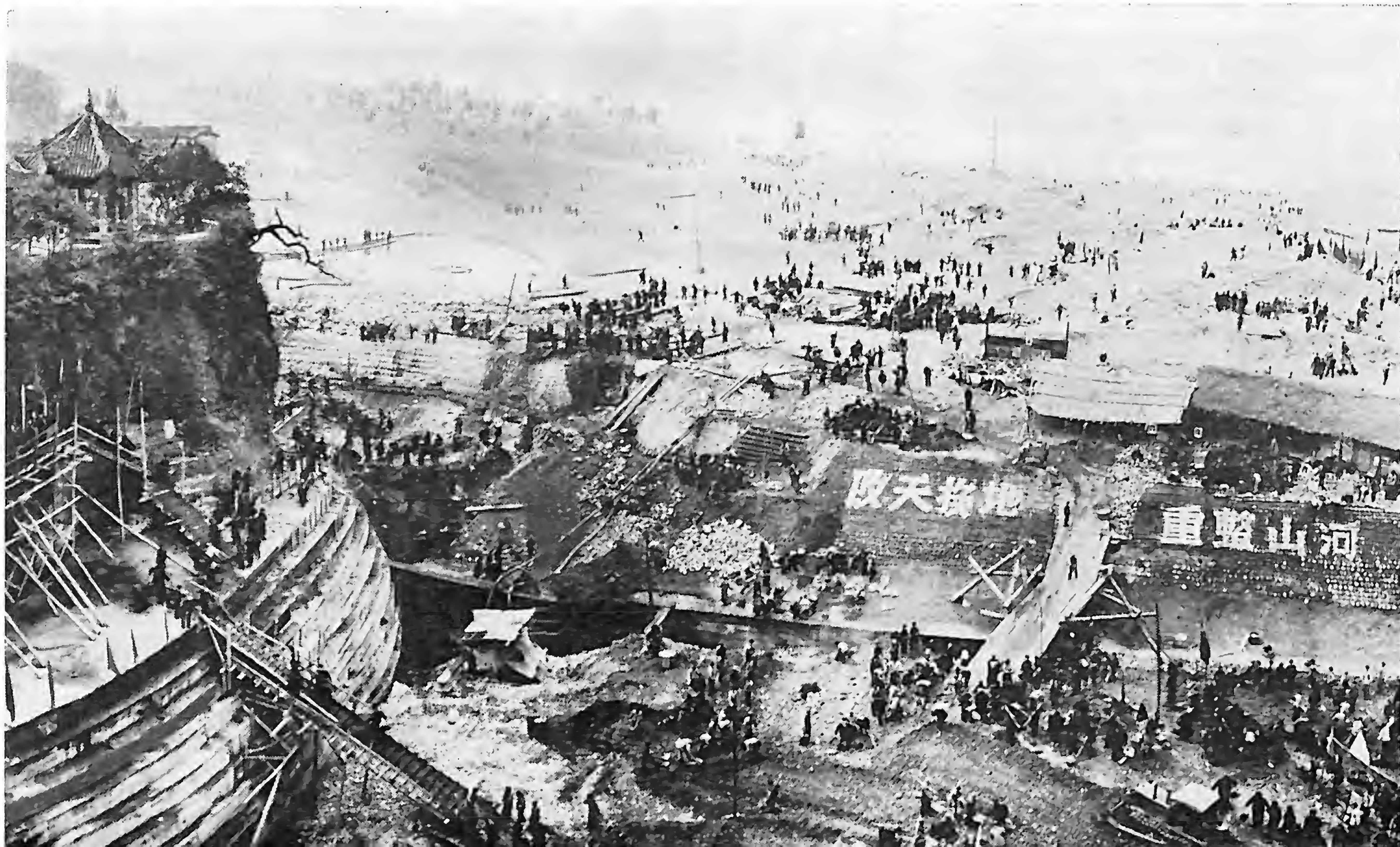
Work proceeds on reinforcing Litui Rock.
